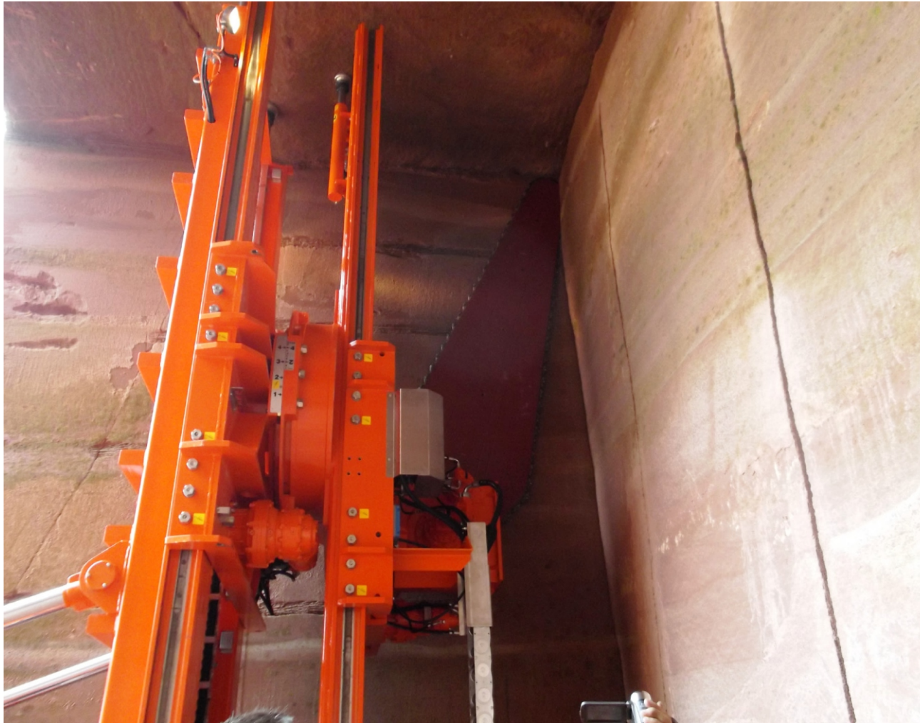
TAGLI VERTICALI A PARETE VERTICAL CUTTING AT WALL SIDE
